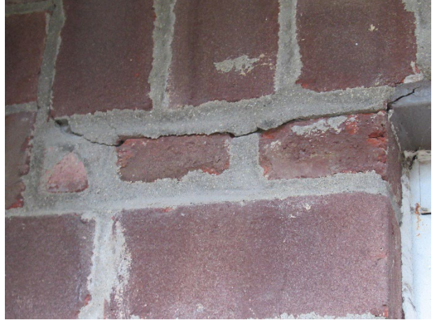
Mortar deterioration
