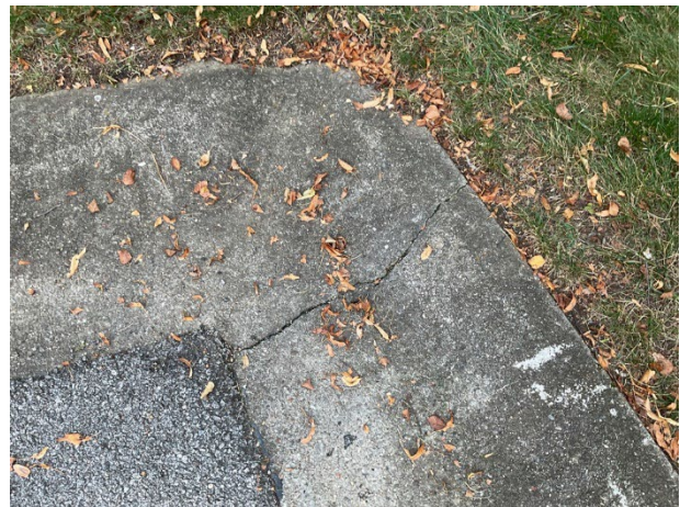
Concrete cracks
