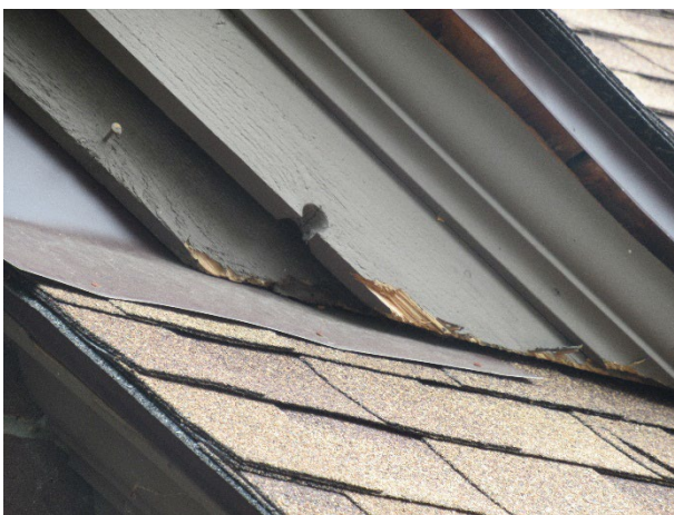
Finish deterioration
