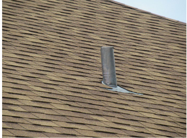
Waste pipe with metal boot
