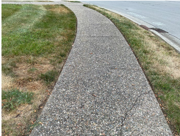
Concrete sidewalk – We note concrete cracks
