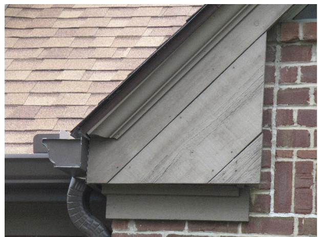
Finish deterioration
