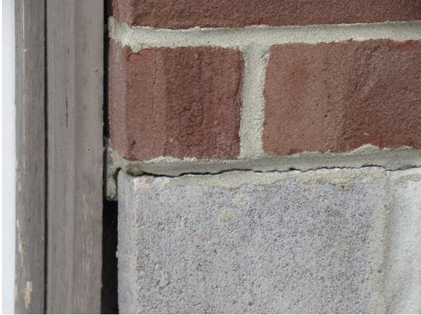
Mortar deterioration
