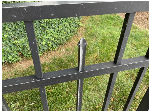
Finish deterioration
