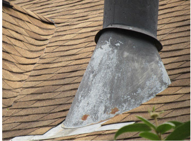
Deterioration on base of chimney cap
