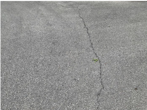
Pavement cracks
