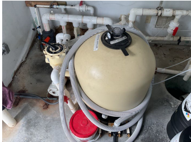
Pool pumps and filters
